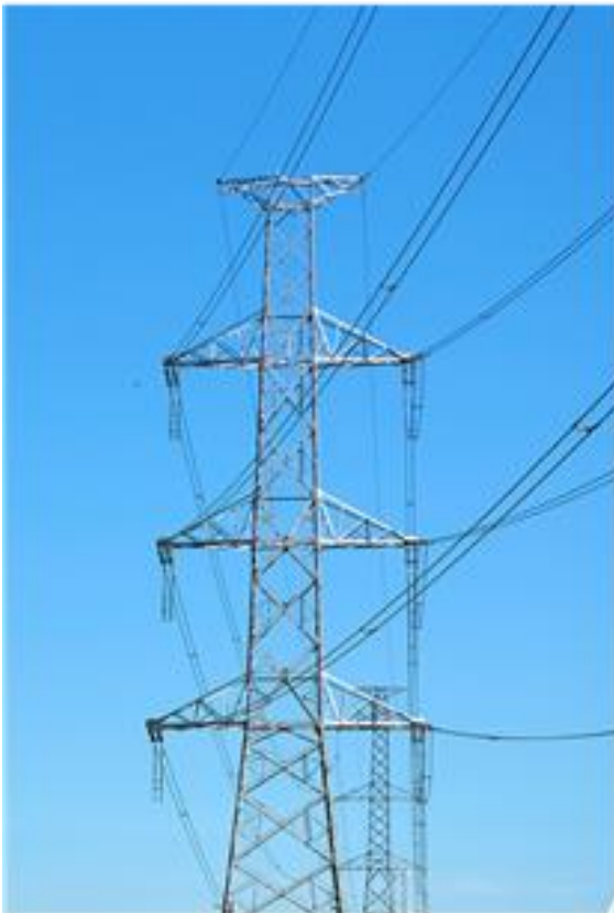
Figure 2: 380 kV steel lattice tower
