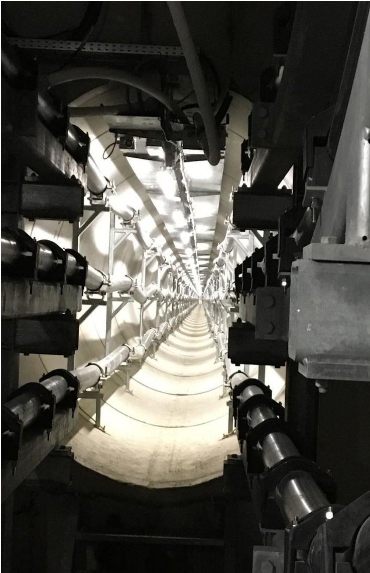
Figure 7: 380 kV cable system tunnel installation
