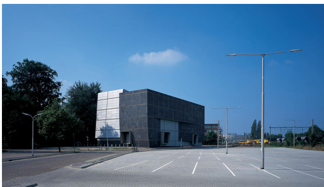
Electricity substation, Amersfoort, Nederland - UNStudio
