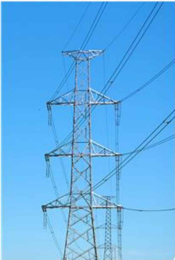
Figure 2: 380 kV steel lattice tower
