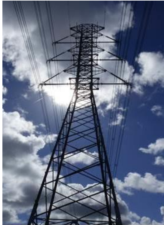
Figure 5: Compact 380 kV tower
