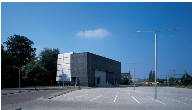
Electricity substation, Amersfoort, Nederland - UNStudio
