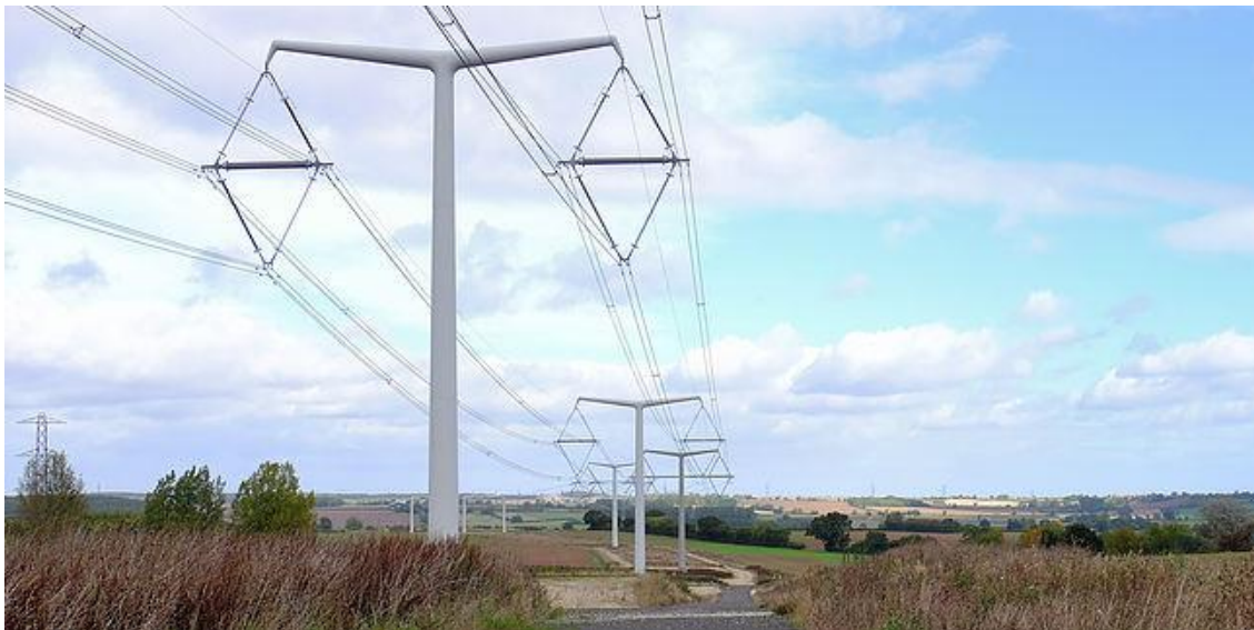
Figure 6: 380 kV folded steel structure
