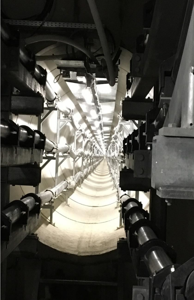
Figure 7: 380 kV cable system tunnel installation
