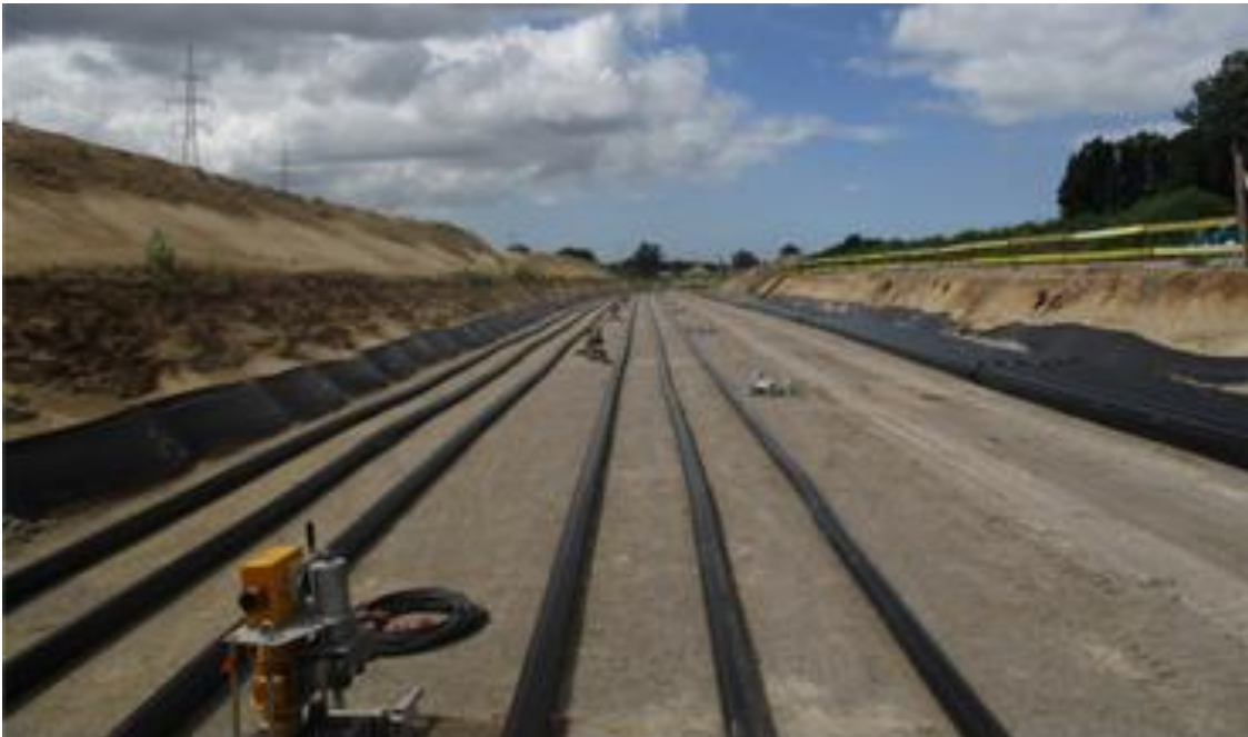
Figure 6: 380 kV direct buried cable circuit prior to backfilling
